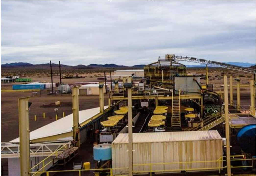
Processing Plant at Copperstone
